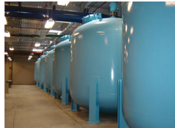
Example Filter Vessels – Westtech
