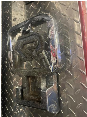
Side Pump Panel Corrosion
